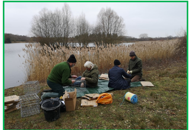
Fish refuge creation: volunteers making steel gabion baskets, January 2023
